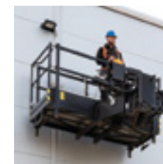
Man platform ready
